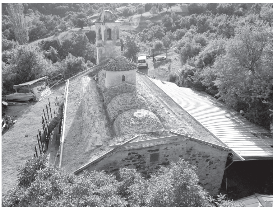
The St. Kyriaki Church in the village of Dokatichevo from above, with the roof structure exposed
